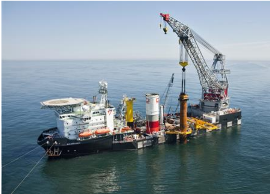
Vibro-pile installation at Riffgat OWT; (RHS) pile head with vibro-driver (Cape Holland)
