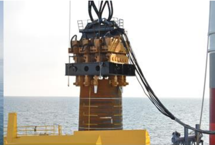
Vibro-pile installation at Riffgat OWT; (RHS) pile head with vibro-driver (Cape Holland)
