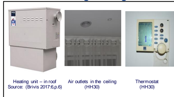
Ducted forced air heating system – through ceiling
