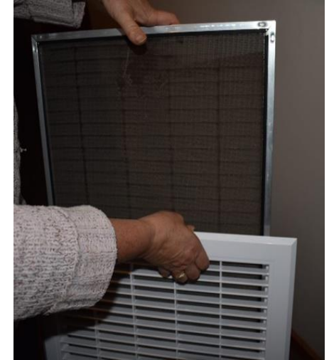
Cleaned return air vent - HH34
